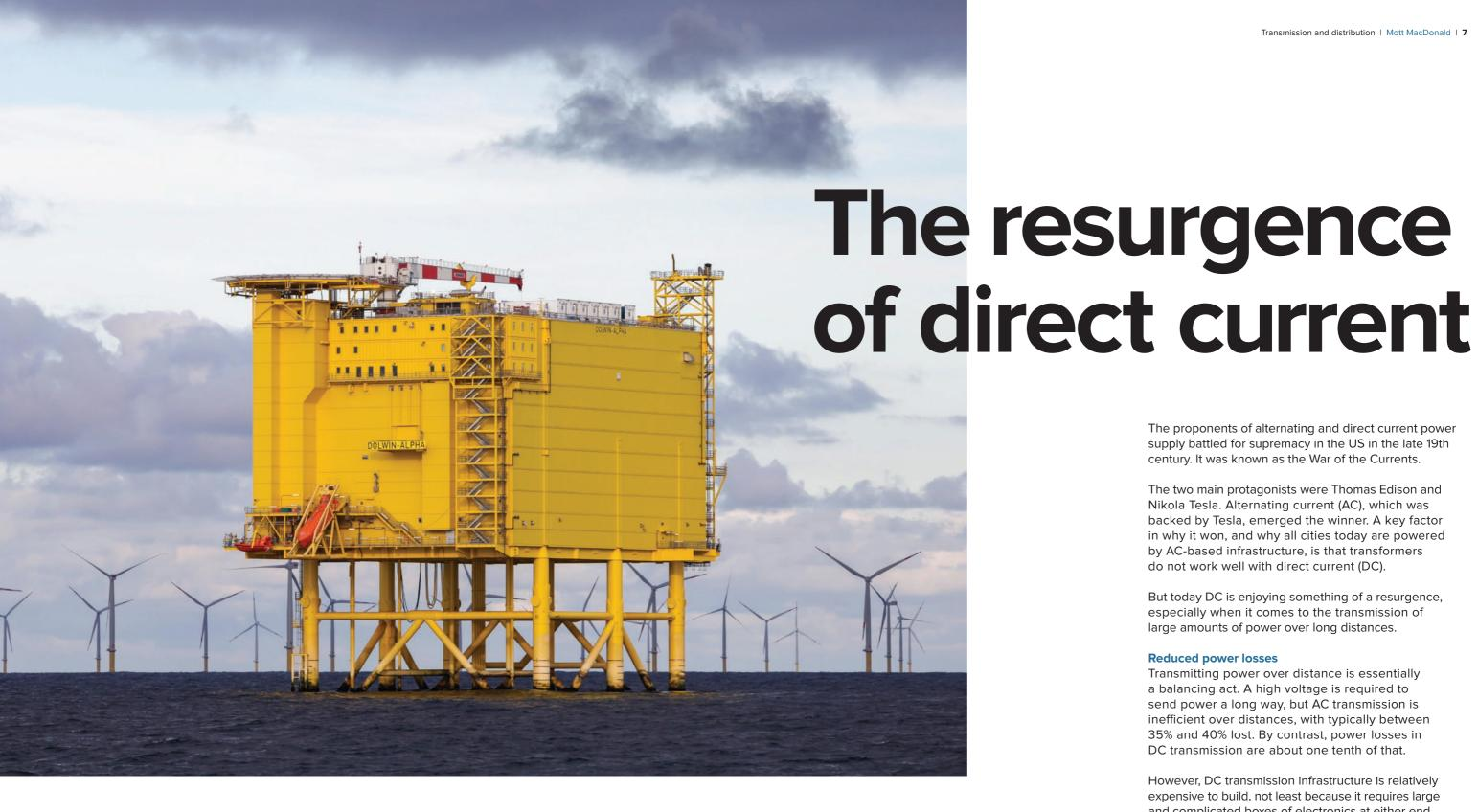
Advances in power electronic converters makes high-voltage direct current feasible for long-distance transmission
